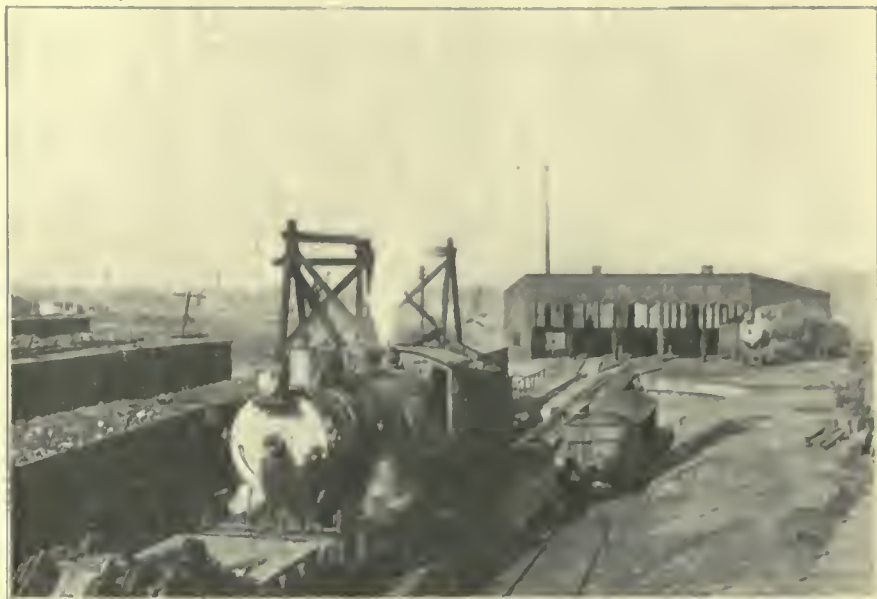
FIG. 678. FACILITIES TO BE REMODELED. View in the HY Tower Yard of the Chesapeake & Ohio Railway of Indiana. Under the proposed plan of electrification, slight changes in the track and building arrangement of this yard will be required. The present engine house will remain as shown and proper buildings for electric locomotives will be added, together with the necessary tracks to accommodate the new service.
